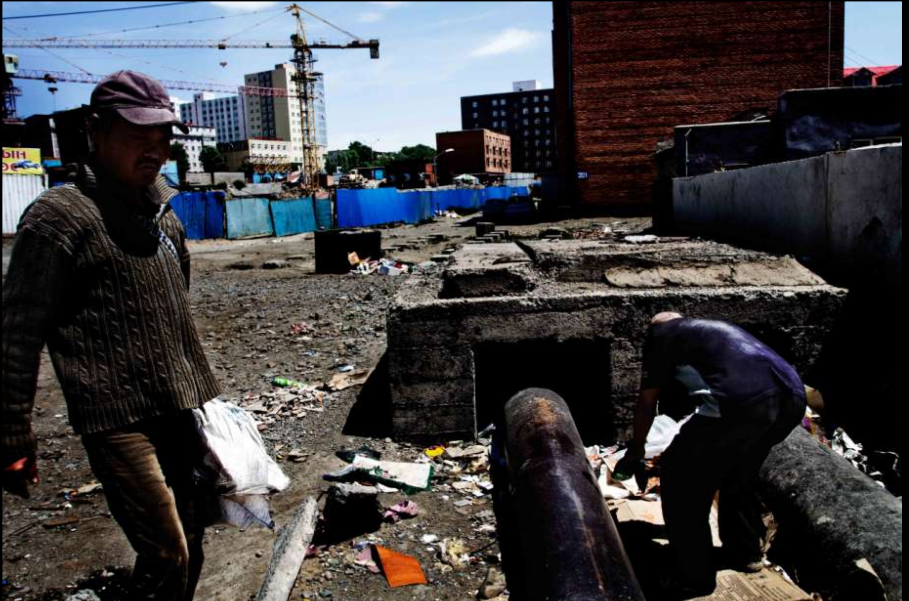
In a building site finding a cleaner and comfortable shelter is easier. Unfortunately this place is not accessible.
